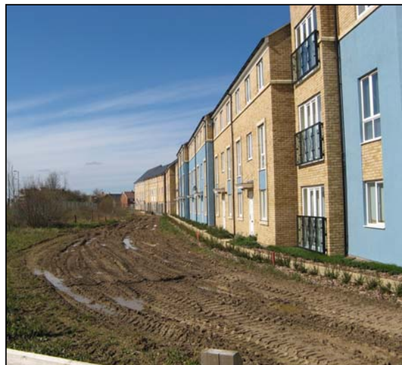
The Cambridgeshire Guided Busway is under construction at Arbury Park
